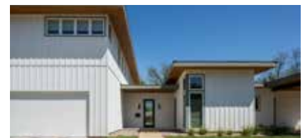
HardiePanel vertical siding with HardieTrim Batten board for the Board & Batten look.
