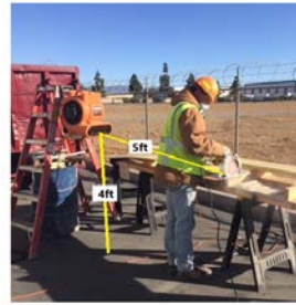
Cut Station Configuration 2
