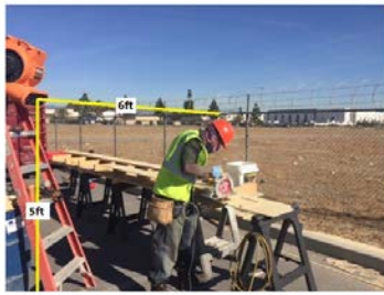
Cut Station Configuration 1
