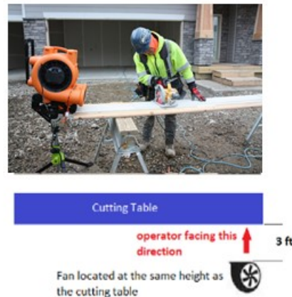
Circular Saw Setup 1
